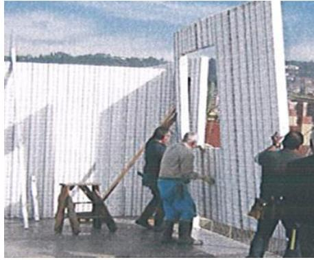
Figure 6. Structural Insulated Panel system (SIP) (foam core sandwiched)
